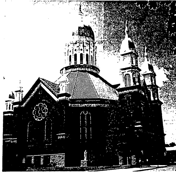
ST. STANISLAUS CHURCH is getting air conditioning, with the mechanical room 85 ft up in the large center dome.
